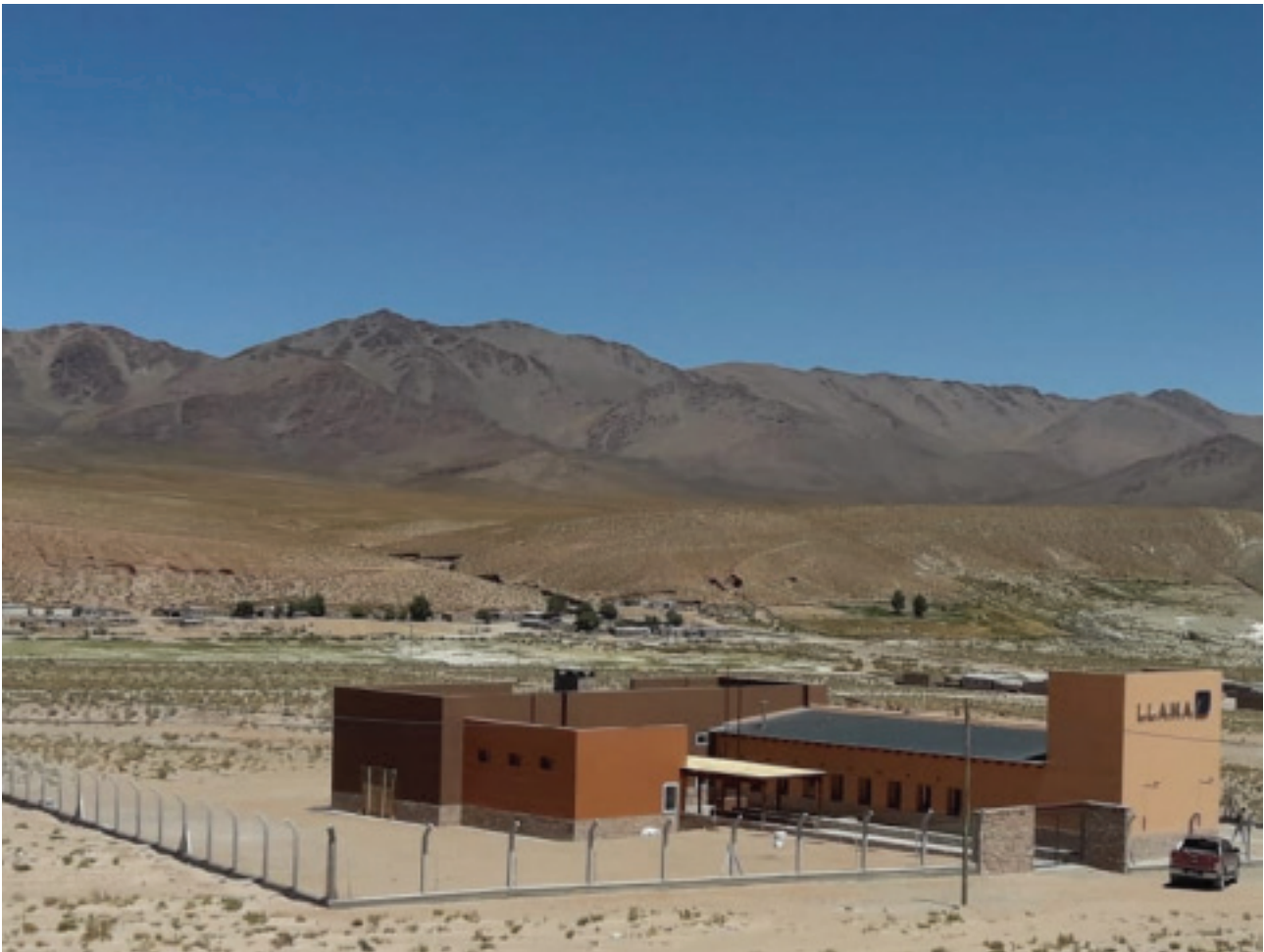
Figure 2. LLAMA building for administration, lodging, and labs in San Antonio de los Cobres, Salta. Credit: Gobierno de la Provincia de Salta.
