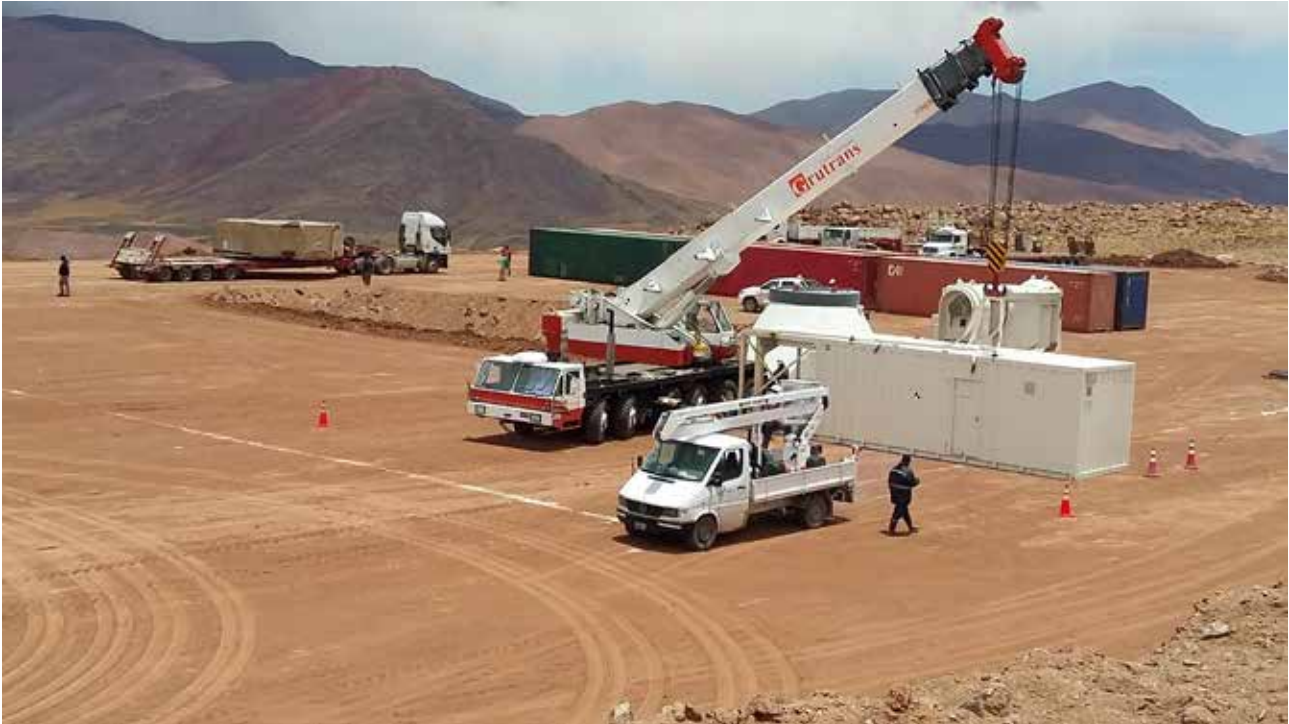
Figure 9. View of the installation of different components of LLAMA antenna in Alto Chorrillos . Credit: Fundación CAPACIT-AR and Instituto Geonorte, INENCO (CONICET).
