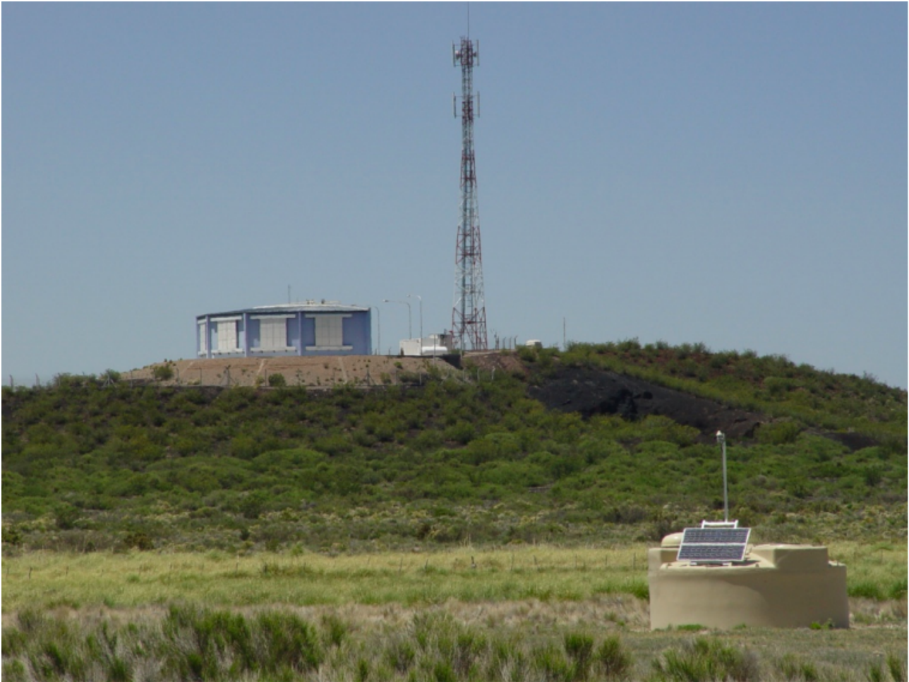
Figure 2. One surface detector deployed in the field, in the background one of the FD buildings and the communications tower.
